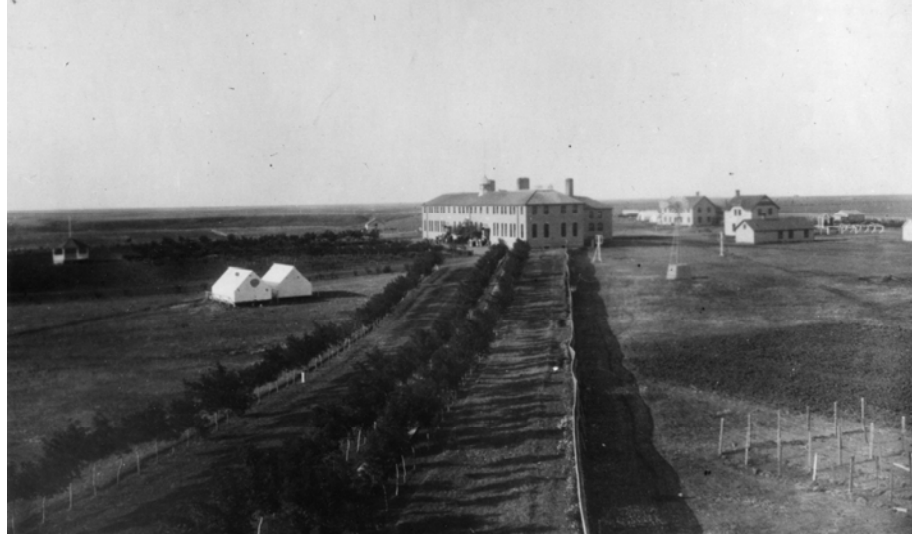
FIGURE 1. Tents erected on the school grounds for students with tubercular and related respiratory conditions. (PAS R-A21262-1)
